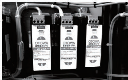
Power line Class I SPD in actual installation
