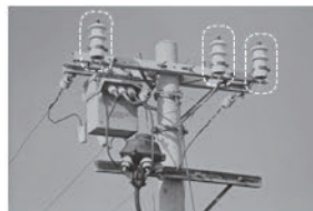
Distribution arrester of early stage (P-Valve Arrester)
